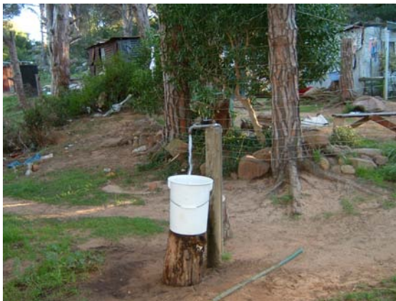
Figure D1.4: Tapstand at Redhill
