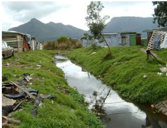
Figure D1.10: Stormwater channel to wetland, Masiphumelele
