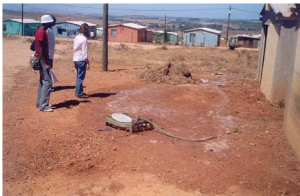
Figure D1.13: Water supply at Lingelethu
