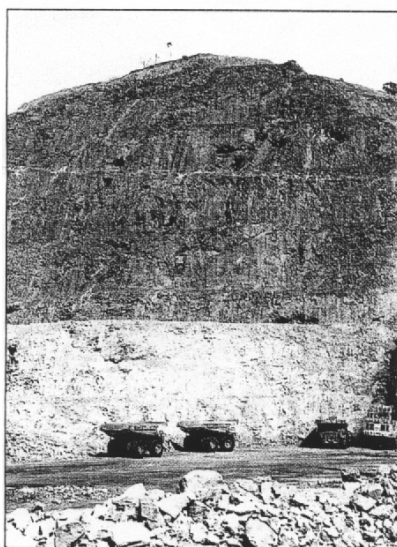
East wall of the Office Pit clearly showing abandoned workings. The Office Pit is part of Kalgoorlie's Fimiston Super Pit.
