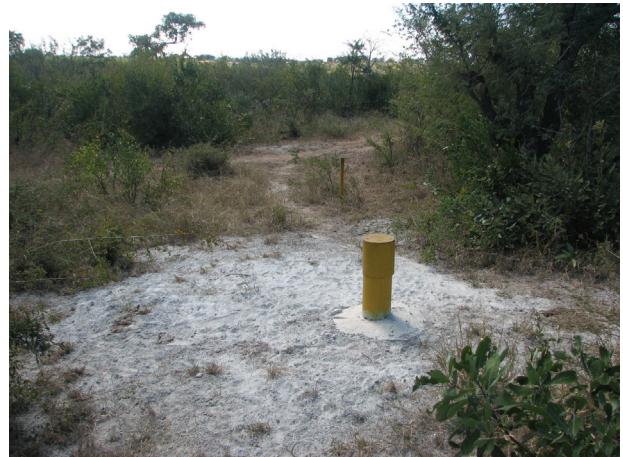
Photo 1. Borehole drilled 72 mbs and 120 mbs in the Hout River and Goudplaats Gneiss in the Limpopo Province respectively.
