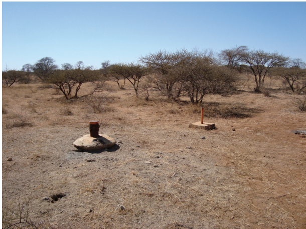
Photo 1. Borehole drilled 72 mbs and 120 mbs in the Hout River and Goudplaats Gneiss in the Limpopo Province respectively.
