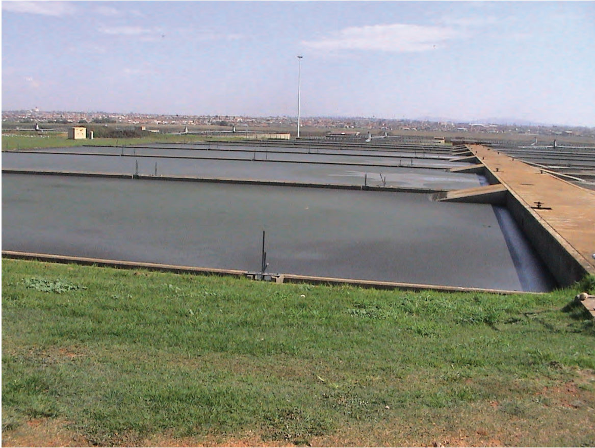
Figure 5.4 Concrete drying beds at Vlakplaas from which sludge was taken for this study
