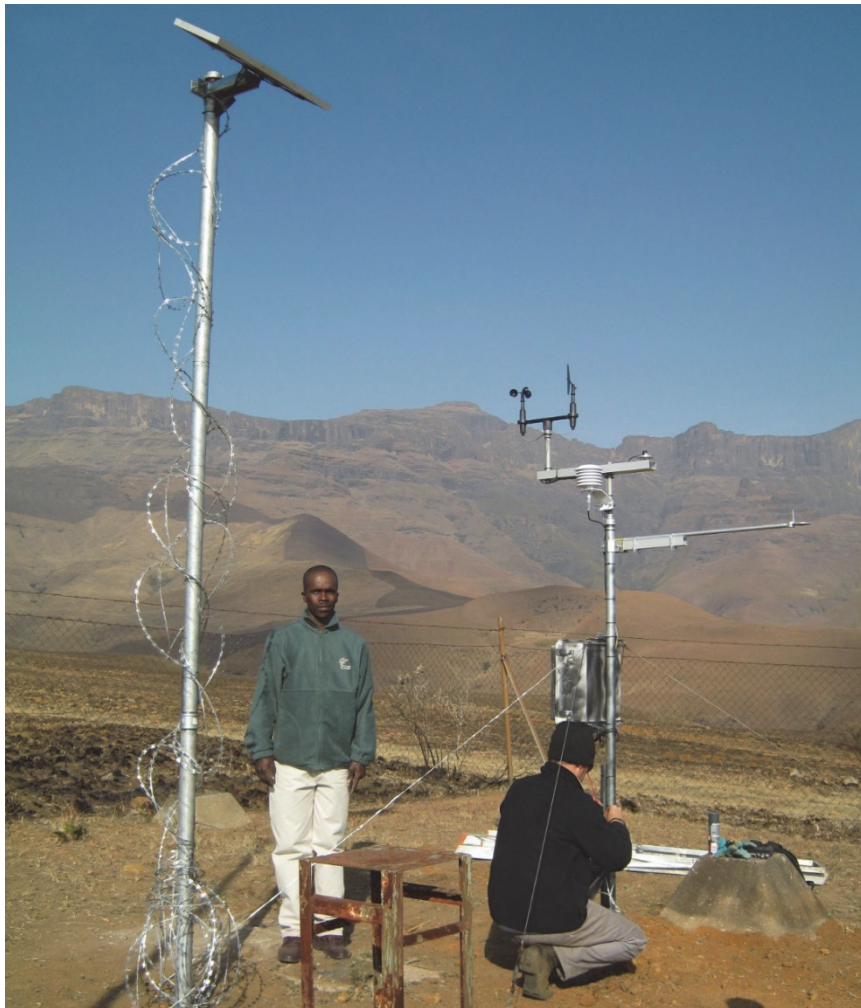
Figure 3.6: Installation of the automatic weather station at Mikes Pass in August 2012
