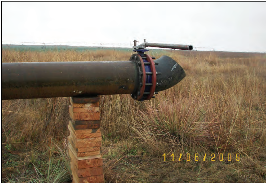
Figure 4-40: Equipment installed to be able to release flow from the B16 pipeline to generate a negative pressure wave
