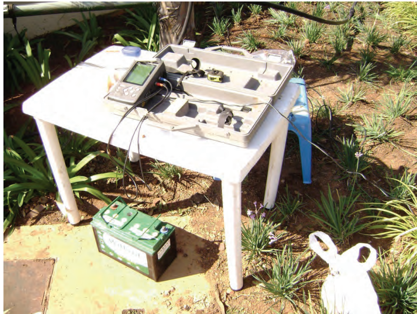
Figure 4-7: Flow recording equipment (Fuji)
