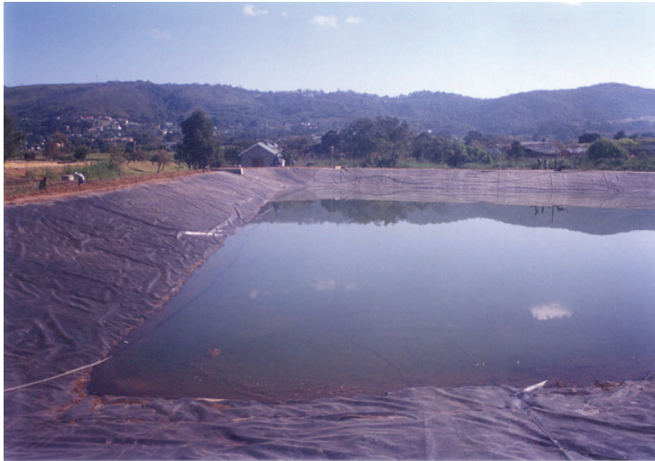
FIGURE 9. LINED EVAPORATION POND
