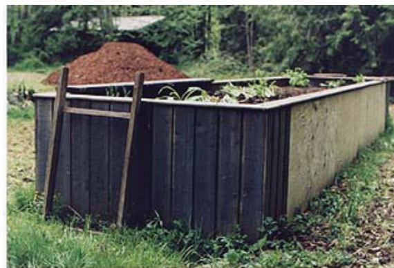
Figure 62: Example of a greywater planter in British Columbia (from http://www.greywater.com ).
