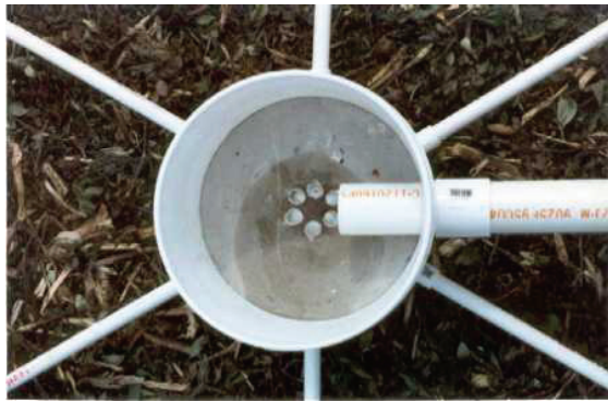
Figure 68: Example of a Casa Juliana greywater treatment and distribution system. A) Grease interceptor. B) Six pipes to distribute greywater. C) Distribution hub. D) Infiltration chamber at the end of a pipe. (From http://www.omick.net .)
