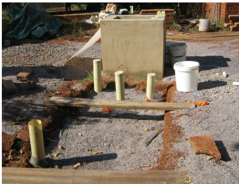
Figure 5: Combination of mulch tower and sub-surface resorption bed, including embedded infiltration zone and surrounding gravel filter. Projecting pipes are access points for sampling.
