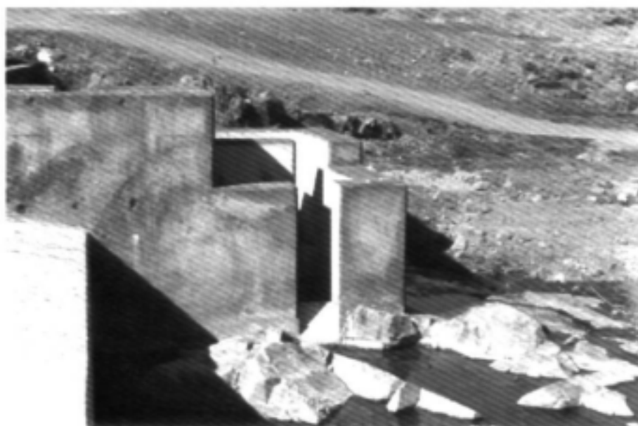
Plate 3.4: View of most downstream slot of the "Pool and Slot" Ten Bosch fishway on the Crocodile River in the KNP, during low stream-flow conditions (no flow through fishway).
