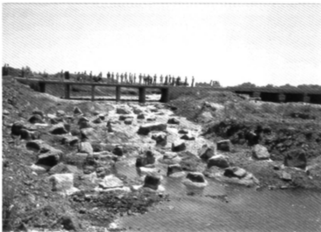
Plate 3.6: Lower Sabie bridge Rock-ramp fishway at commissioning in October 2001.
