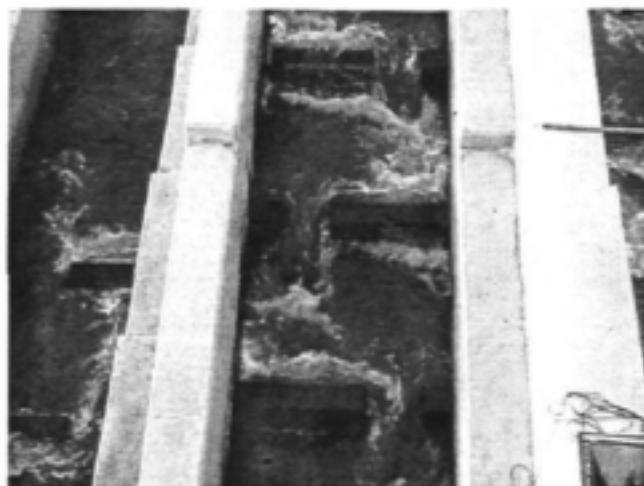
Plate 8.3: Flow pattern in the fishway
