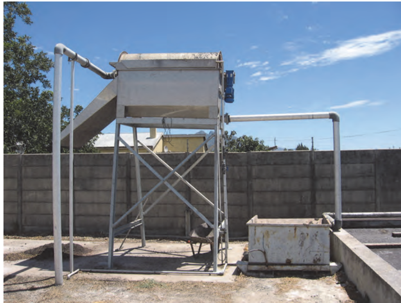
Figure 2.4. Screening equipment used to remove coarse particles from the winery wastewater.
