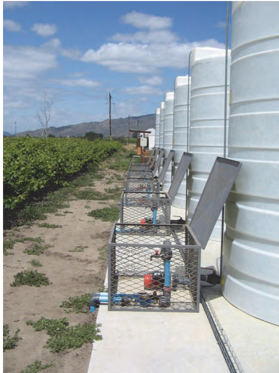
Figure 2.3. Tanks in which winery wastewater was augmented with raw river water before it was pumped to the different treatment plots.
