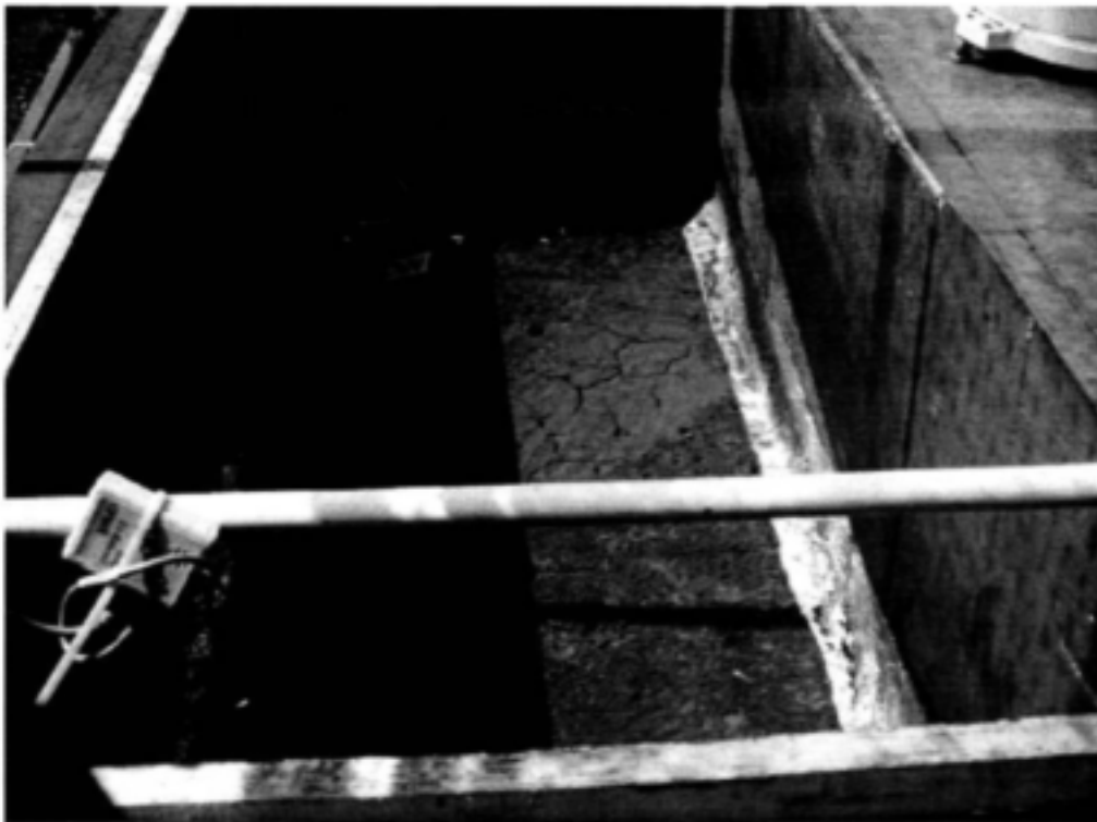
Figure 24: Cracks evident on the surface of the soil material after wetting events
