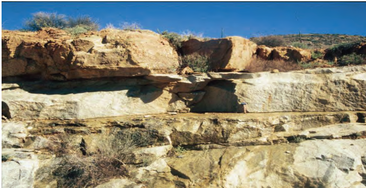
Figure 27: Water flowing from regularly spaced horizontal joint planes. The surface planes of the vertical joints are clearly visible.
