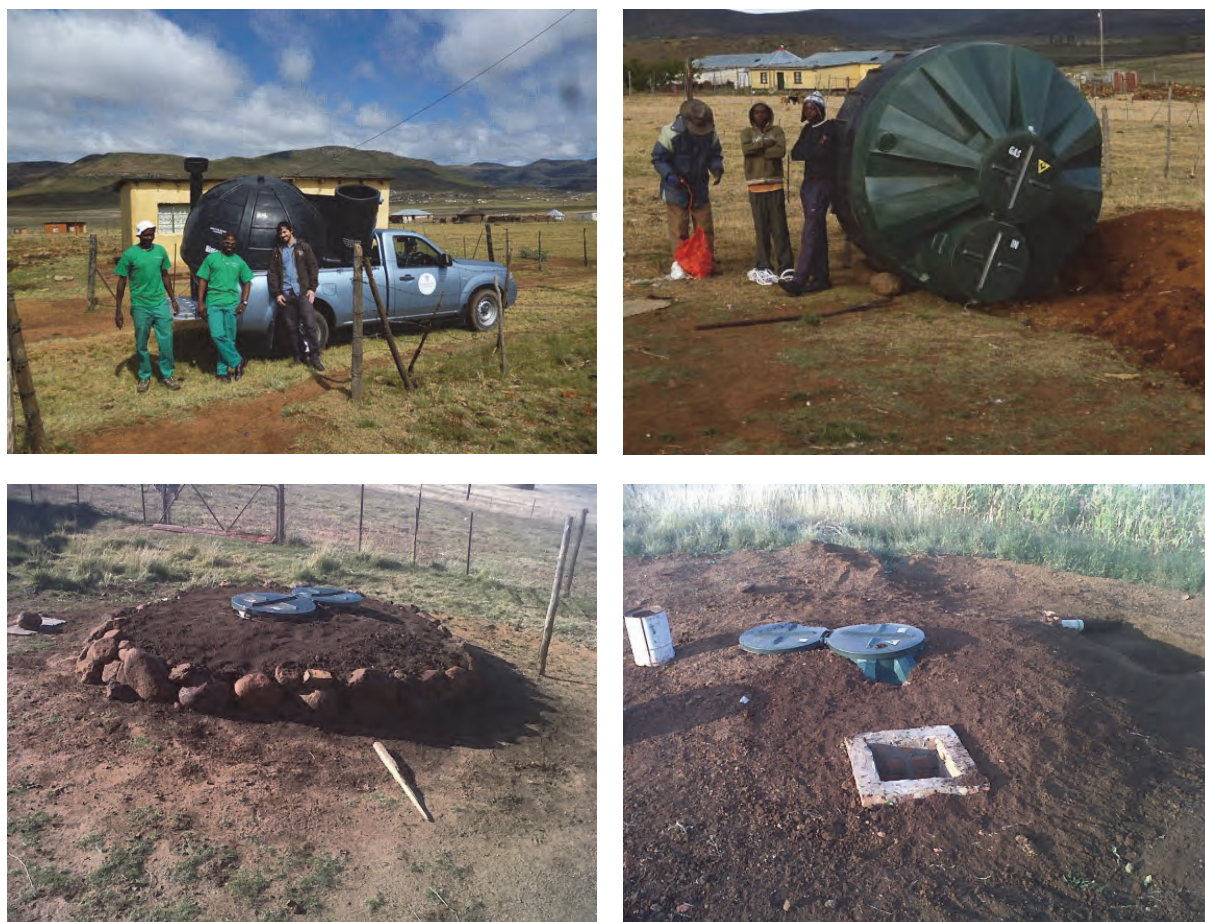
Plate 4.5: Clockwise from top left: (a) Biogas Pro digester before installation (b) Biogas Pro digester installed and insulated (c) Indian Sintex before installation and (d) Moisture trap (brick structure in foreground) in relation to biodigester.
