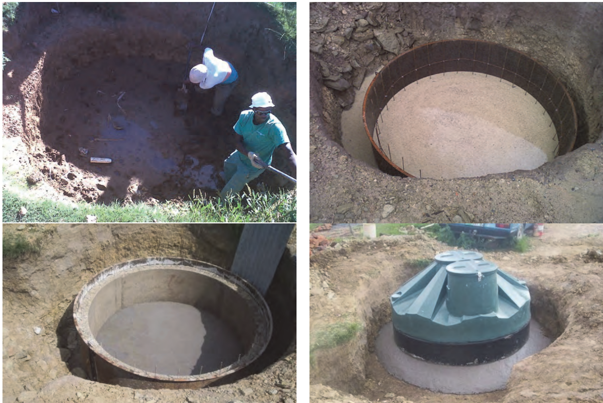
Plate 4.6: Clockwise from top left: (a) expanding the initial hole due to collapse, (b) flooding of the site, (c) concrete frame completed (d) final view before coverage.
