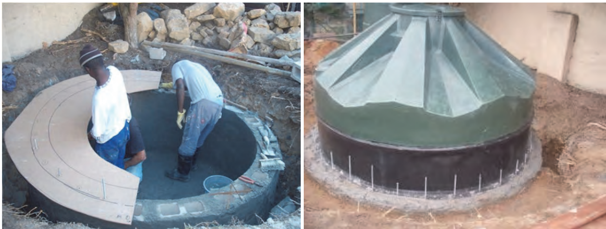
Plate 2.2: A BiogasPro SmartTop digester being installed, the base of tank is built on site (left), the SmartTop is installed and sealed onto the unit (right).
