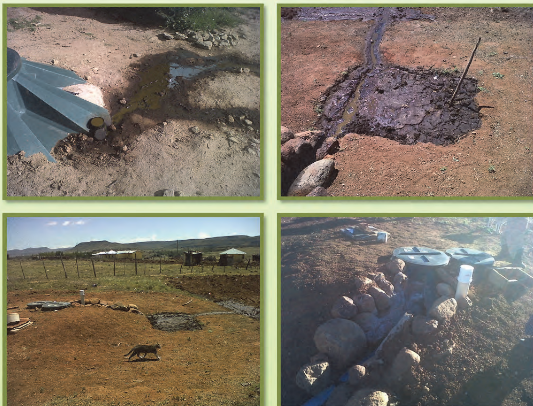
Plate 6.4: Clockwise from top left: (a) Initial outflow pipe, with no bioslurry retention capacity, (b) evidence of slurry accumulation, (c) biodigester location in relation to field, and (d) new outlet constructed using rocks and cement to increase slope and ensure no backflow.
