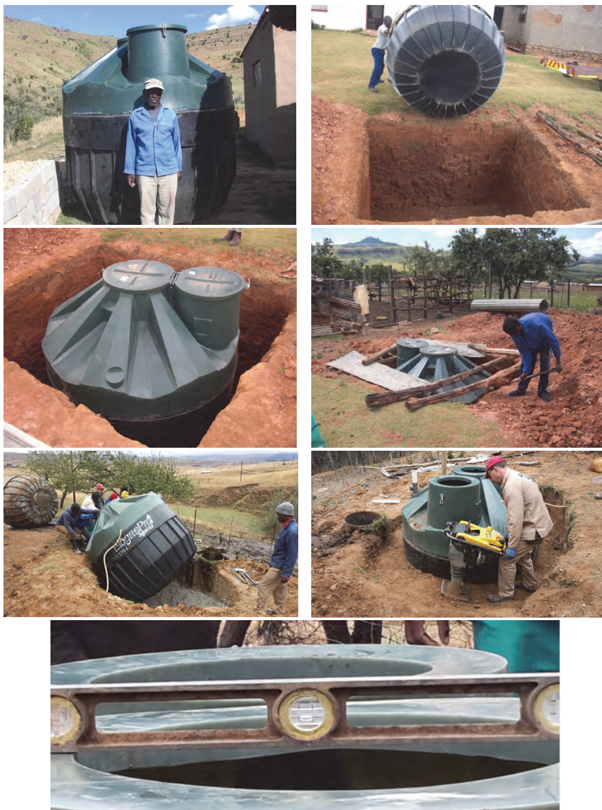
Plate 4.2: Installation of biodigesters in KZN.
