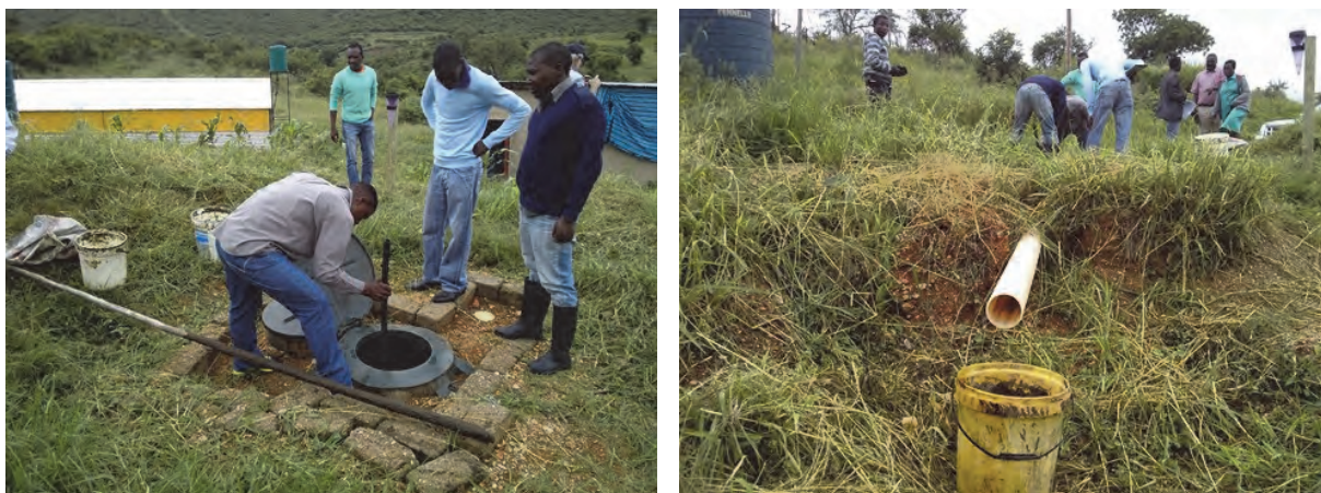
Plate 4.7: Pictures showing the biodigester and slurry outlet pipe installed at Nthabalala.
