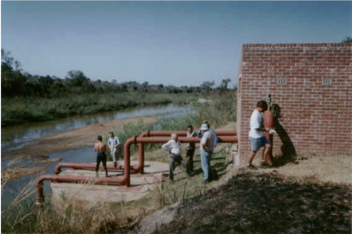
Figure 1.1: Sand River water intake structure and pumphouse with suction pipelines on riverbank. Extensive sandbanks in the river course are visible in the background.
