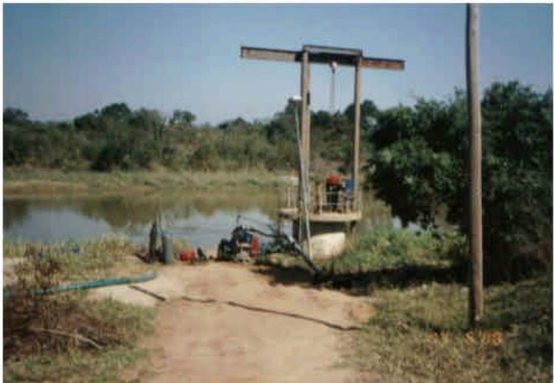
Figure 5.5 : Thulamahashe Intake on a tributary of the Sabie River
