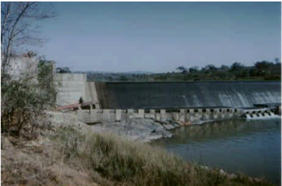
Figure 5.7 : Dwarsloop intake (intake pipe is visible on left side where it passes through the weir at a relatively low elevation)
