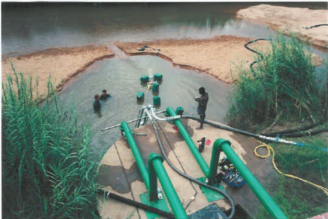
Figure 7.2 : Dredging of a crater by means of the mobile trailer unit in progress at the Sand River Intake
