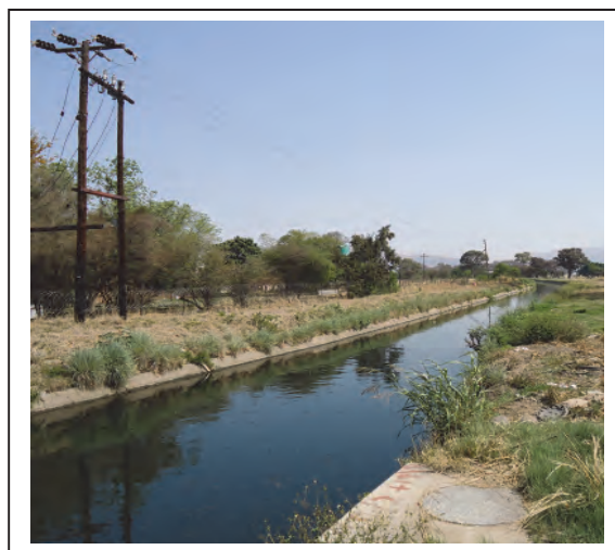
Figure 46: Large capacity canal in Madibeng for irrigation
