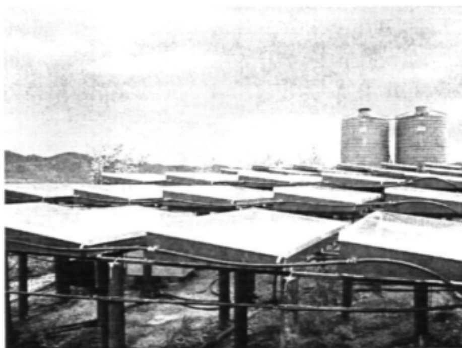
Figure 7: DWAF solar still plant at Algerynskraal in the Klein Karoo with Solardome-manufactured solar stills.
