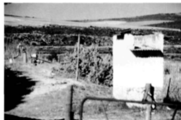
A borehole (blue pipe) sited dangerously close to a pit latrine
