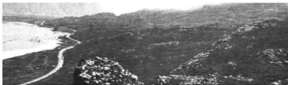
Figure 2.23 Moderate slope near the Theewaterskloof Dam
