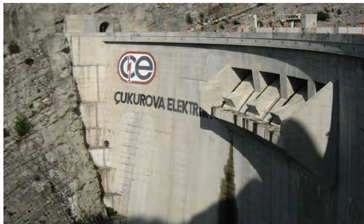
Figure 4.12: Berke arch dam
