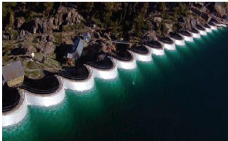
Figure 4.13: Gem Lake dam
