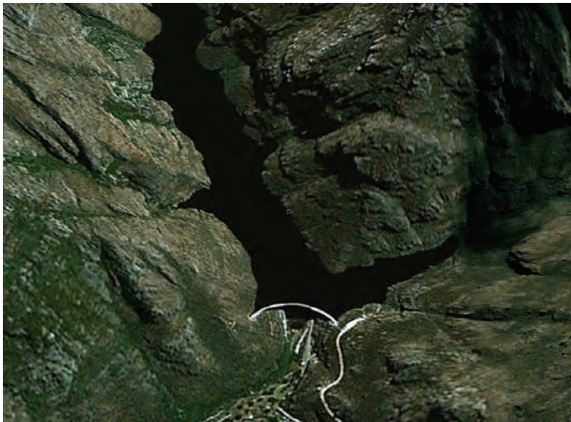
Figure 7.19: An aerial photograph of Roode Elsberg Dam (Courtesy of Google maps, 2005).
