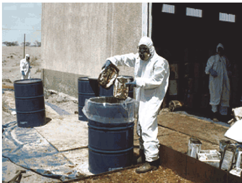
Figure 4-4: A typical clean-up operation for obsolete pesticides showing re-packaging of pesticides for disposal.
