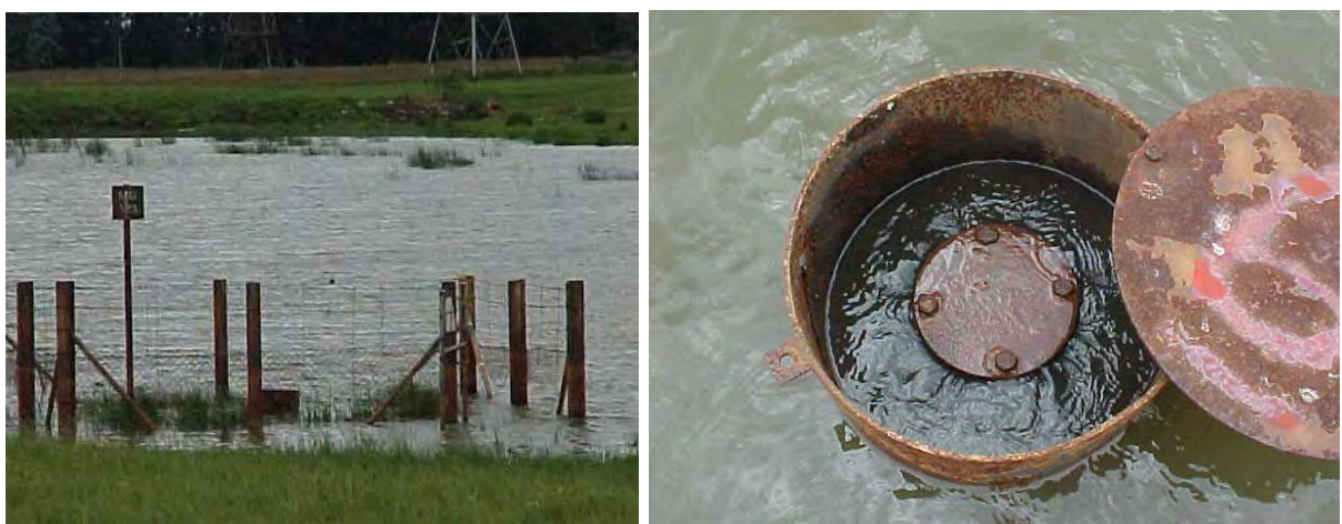
Figure 64. Dam with surface run-off and recharge borehole from the dam into the mine
