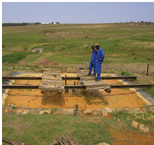
Figure C-2: Temporary wooden deck constructed to enable sampling in centre of SSRU1. (SSRU1 was covered with a bright orange chemical sludge.)
