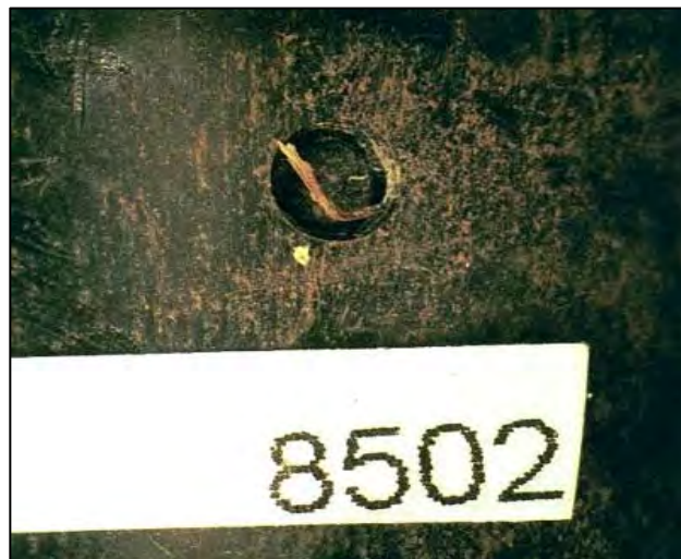
Figure 51: Root in aperture
