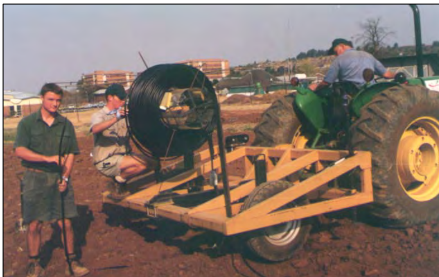
Figure 59: Example of lateral installation implement, as used at experimental site
