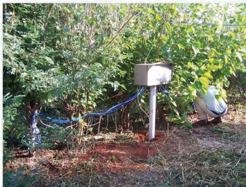
Plate 8.4 The HPV installation in the mature Gleditsia and Mulberry trees at the Mahlobo agroforestry site.
