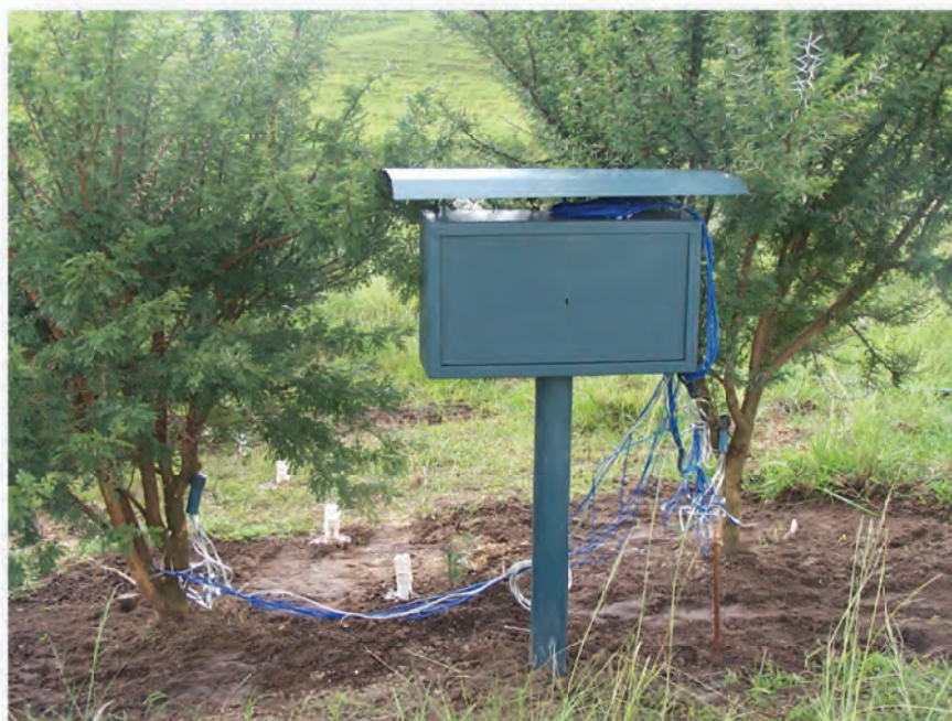
Plate 8.2 The HPV installation in two young Acacia karroo trees at Zwelisha. Note the Diviner 2000 access tubes for soil water monitoring in the background
