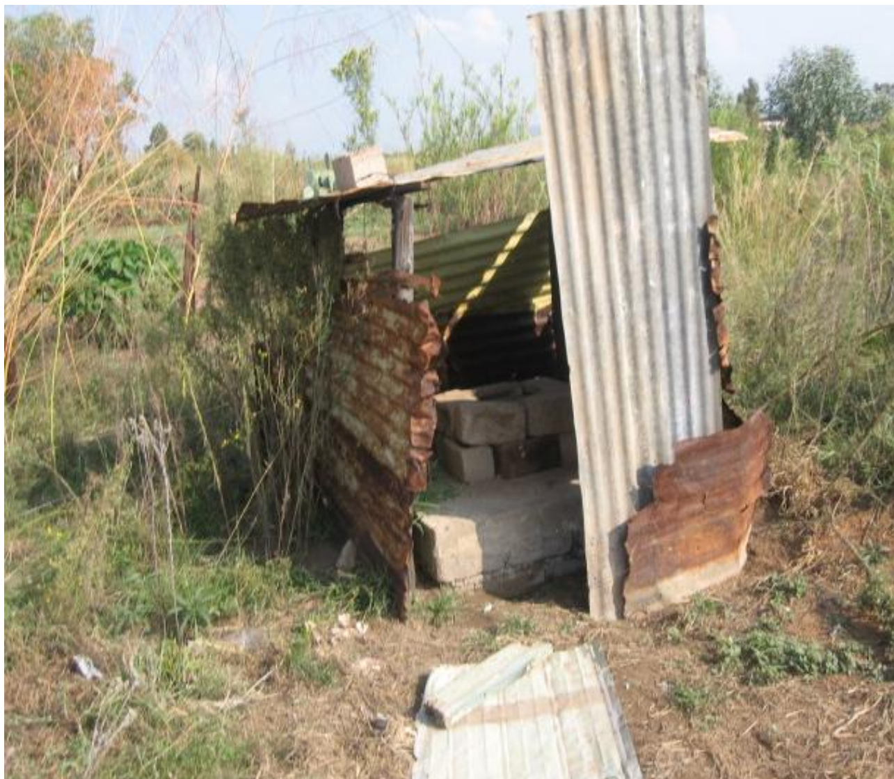
A pit latrine in rural Elansddorn municipality, Limpopo
