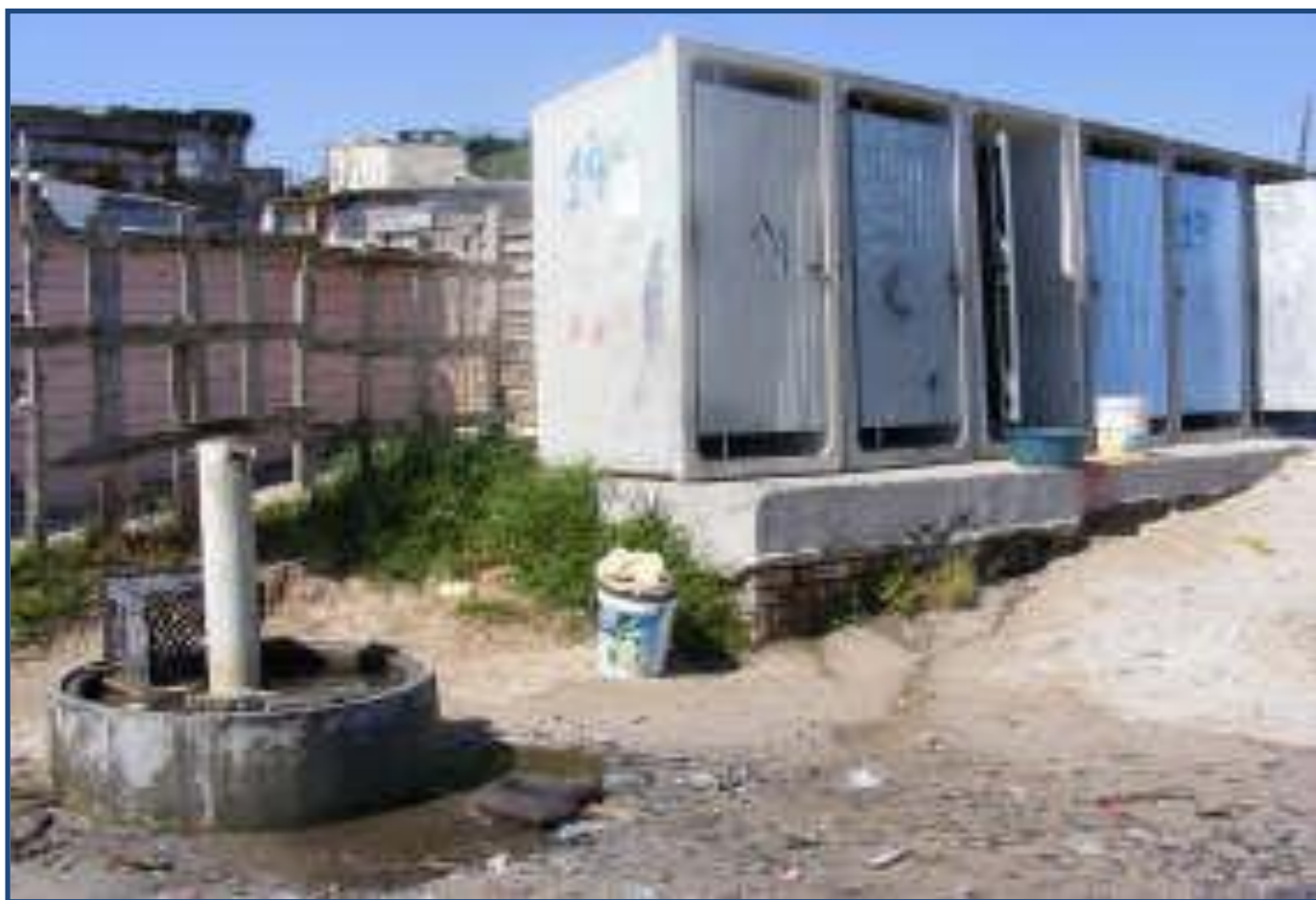
A common water tap next to a block of toilets in Khayelitsha
