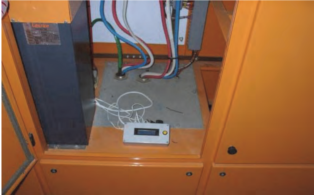
Picture 7: Prototype meter for larger installations (> 50 kW): CTr's outside meter
