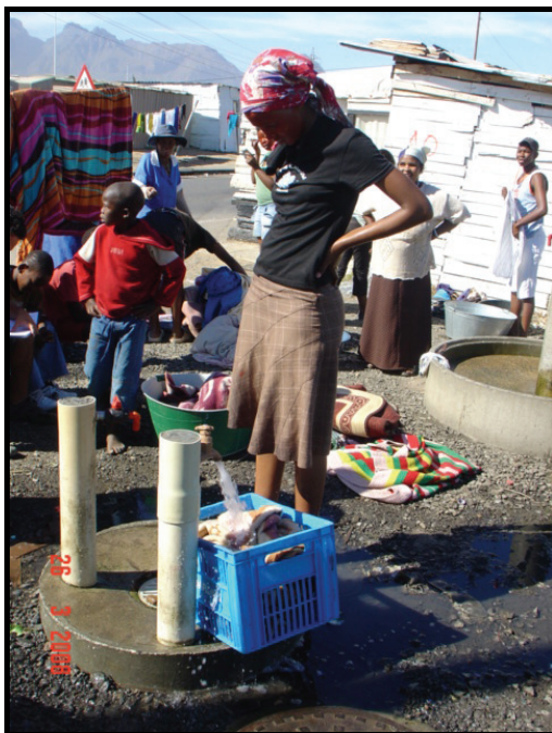
Useful way to rinse washing using open crate placed on raised pedestal. However, excess water does not flow into catchpit but creates wet, uncomfortable conditions surrounding tap. Water conservation is an issue.
