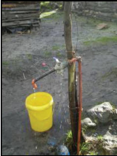
Makeshift and fragile. Inadequate drainage causes streams to flow between shacks.
