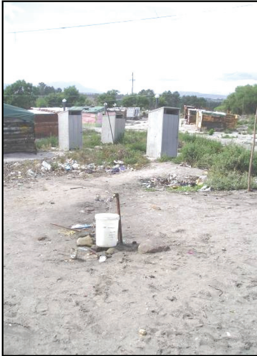
Figure 5.11: A typical tapstand in Waterworks with chemical toilets in the background
