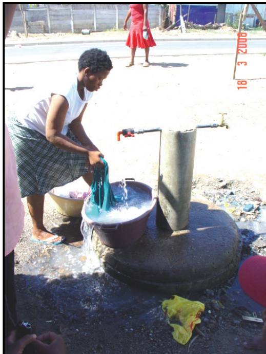
Figure 5.21: Tapstands in Drommedaris showing poor drainage
