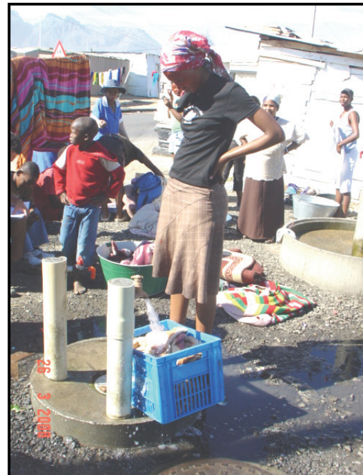
Figure 5.21: Tapstands in Drommedaris showing poor drainage
