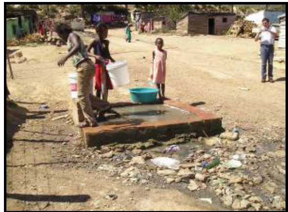
Poor drainage. Catch pit is blocked. Dirty water remains in enclosure.
