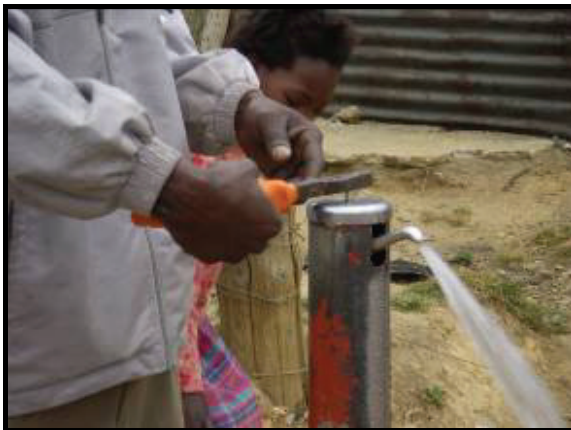
No tap head, but a pair of pliers from a neighbour's house works well.
