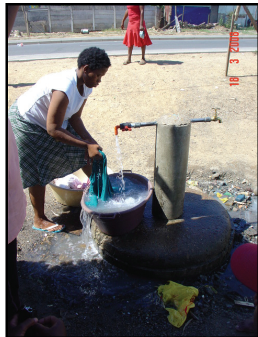
Tap protrudes 30cm from support structure to make it easier for resident to use large basin without spilling water.
