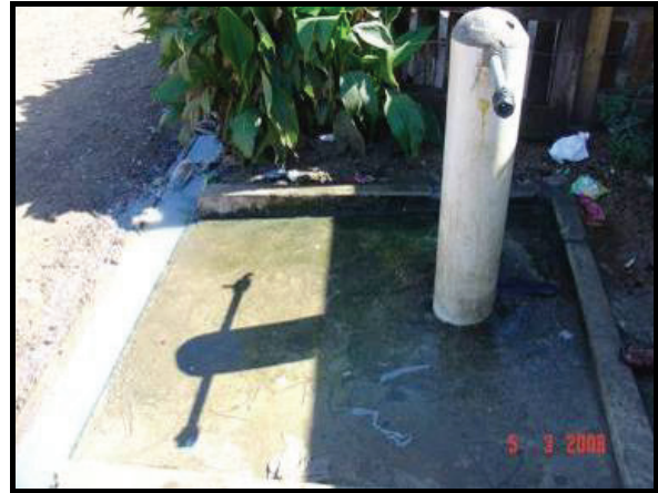
Tapstand catchment allows water to flow along gently sloping hardened surface into open furrow.
