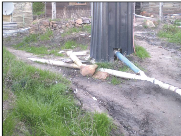
Figure 5.13: A connection to the shallow sewer system
