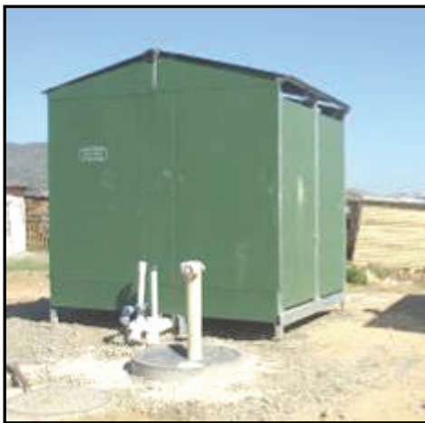
Figure 5.17: Standard tapstand adjacent to AACT ablution block
