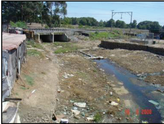
Figure 5.15: Cut-off trench in the river to divert polluted water to the WWTW
