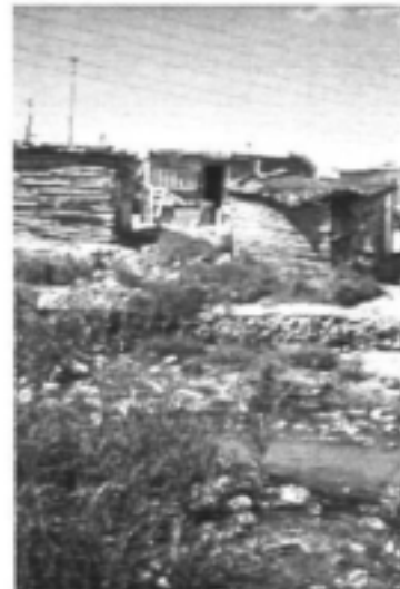
Figure D1.12: Stormwater channel
