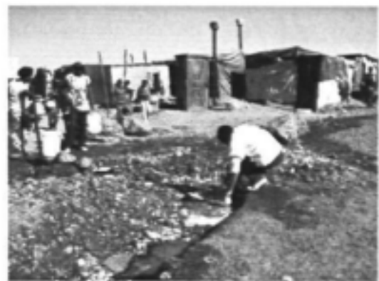
Figure D6.4: Stormwater drain at Freedom Square
