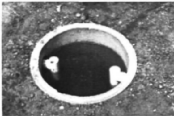
Figure B17.1: Grease interceptor
