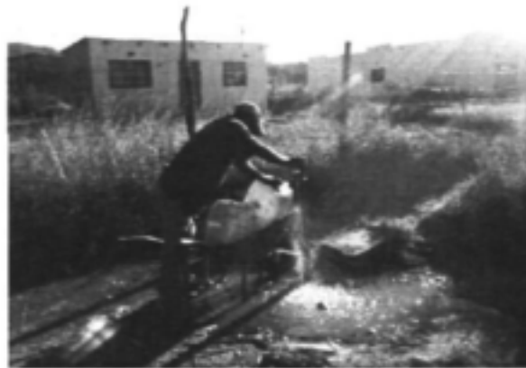
Figure D2.6: Flooded tapstand at Emahobeni
