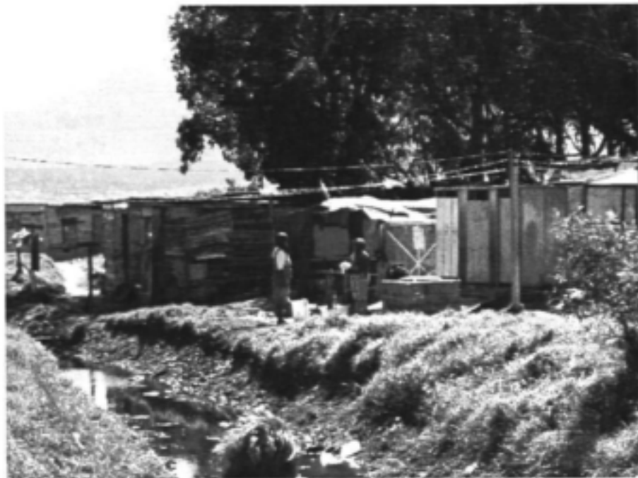
Figure 4.5.5: Tapstand and toilets at Masiphumelele
