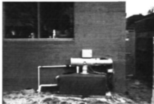
Figure B15.1: Example of Wattworks installation
