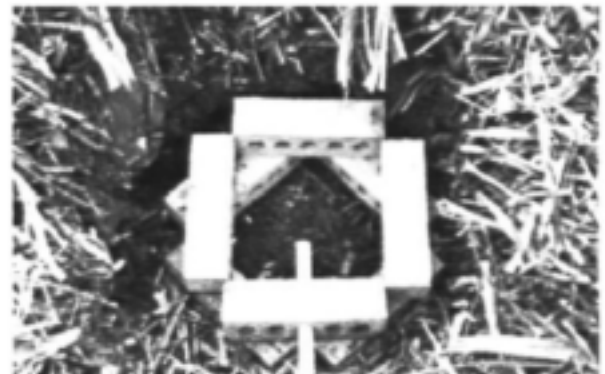
Figure B17.4: Detail of infiltration chamber at end of pipes
