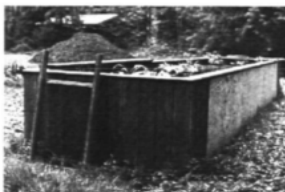
Figure B10.2: Greywater planter in British Columbia
