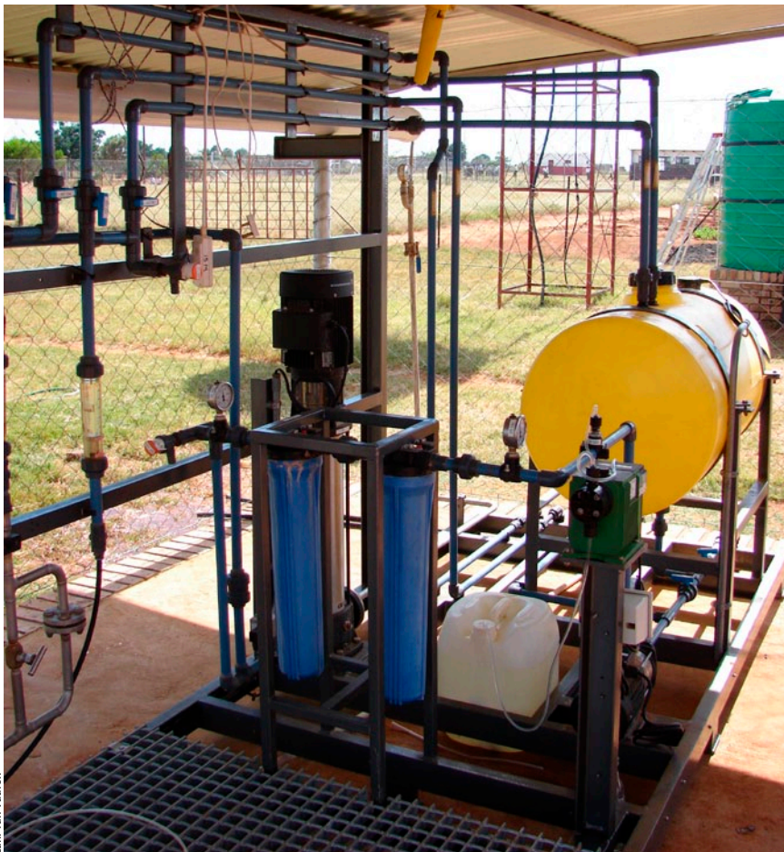
Small desalination plants, such as this one at Madibogo, in North West, are used to treat brackish groundwater for rural communities.
