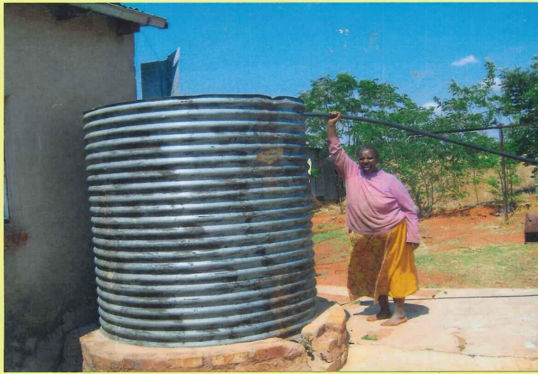
Roof-water System (Collection of rainwater)
