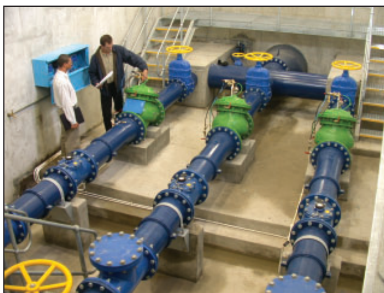
Inside the Khayelitsha water pressure management and control chamber.
