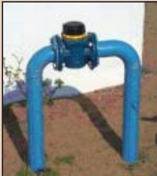
Insufficient straight pipe - perfect air trap
