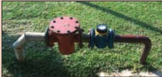
Dirt box too close to the meter
