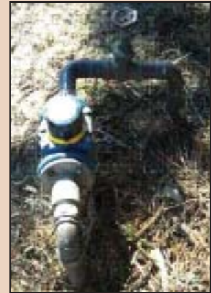
A very poor installation - bends in both the horizontal and vertical plane
