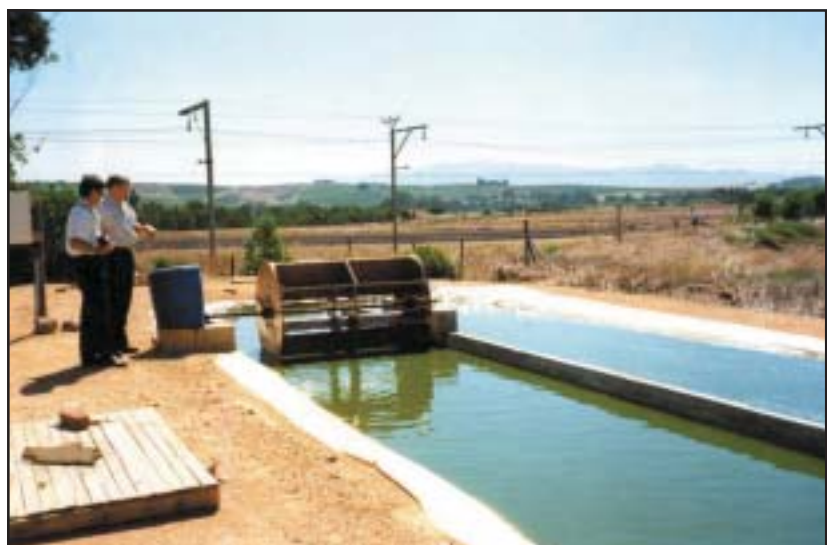
The pilot plant at Wellington featured high rate algal ponds scaled down to 80 m 2 (just under one third of the size of the full-sized operational pond).
