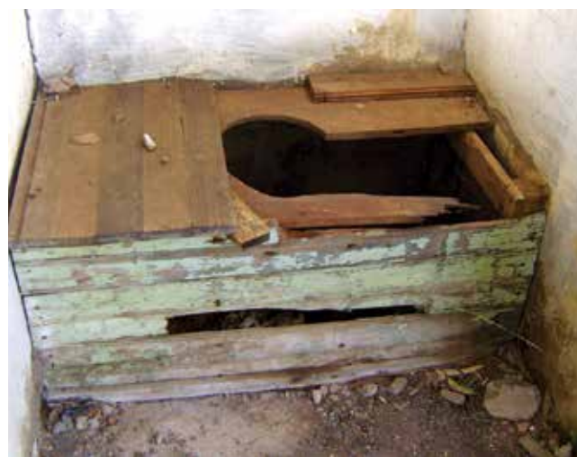
Broken pedestals over pit toilets cause dangerous conditions for learners, especially those in primary school.
