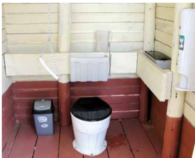
The WRC is funding a project to construct pour flush toilets at six Limpopo primary and secondary schools. The toilets are housed in timber frame units, with the timber coming from removed alien invasive vegetation.
