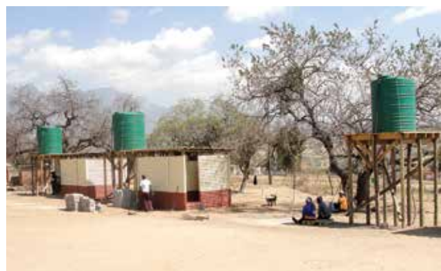
The WRC is funding a project to construct pour flush toilets at six Limpopo primary and secondary schools. The toilets are housed in timber frame units, with the timber coming from removed alien invasive vegetation.
