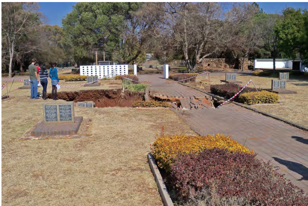
At this cemetery in Irene another issue is clear, namely the formation of a sinkhole that is already an indication of concentrated water inflow in the sub-surface.
