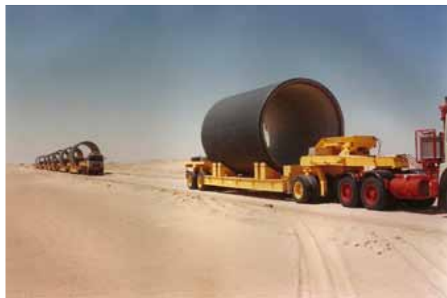
Segments of the massive concrete pipes that were laid to form the man-made river.
