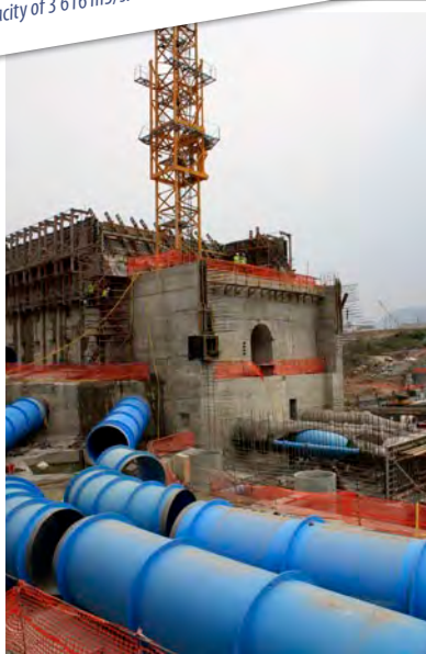
The enormous 2 m-diameter stainless steel outlet pipes. All the pipes are being manufactured at the DWA Central Construction workshops in Jan Kempdorp.
