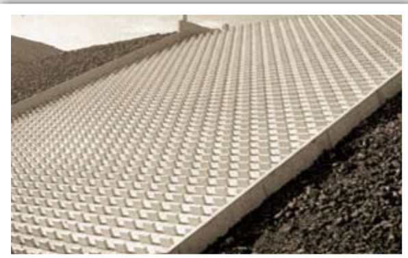
Driekloof Dam features a concrete spillway slab with multiple baffles on the downstream slope.
