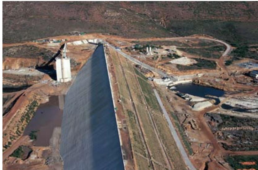
*The Berg River Dam is a concrete-face-rockfill dam type. The dam is 65 m high, 990 m wide and 220 m in width. The gross storage capacity of the dam is 130 million m<sup>3</sup>. The outlet works have been designed to release both low flows and high flows with provision for a peak release of up to 200 m<sup>3</sup>/s. This makes it the first dam in South Africa in which provision is made for flood releases for environmental purposes.*
