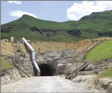
Entrance to the 5 m x 5 m exploration tunnel. The 6 m<sup>3</sup> dump trucks used at present will later make way for articulated dump trucks once construction of the main machine hall starts. Passing bays are being excavated every 100 m along the tunnel to permit empty trucks give way to fully laden trucks hauling uphill.
