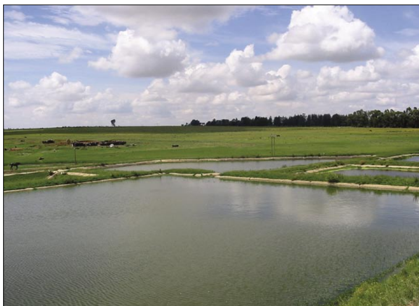
When maintained properly oxidation ponds are acceptable low unit cost ways of treating domestic sewage.
