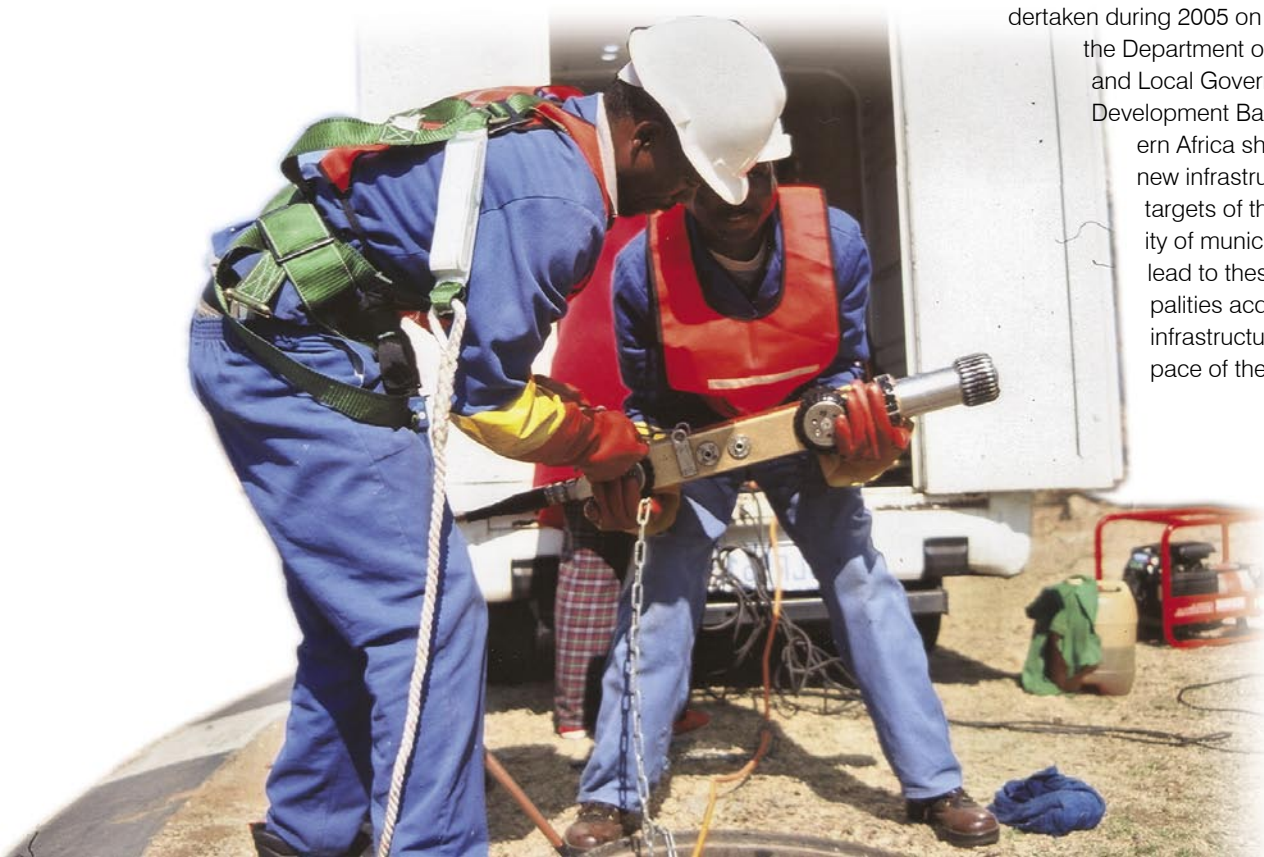
Routine maintenance of sewers is essential to reduce sewage spills.
