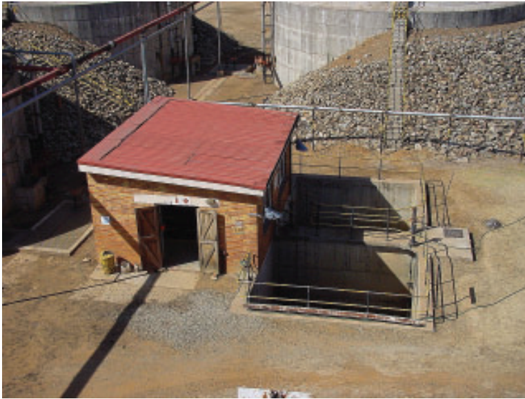
The Ancor sludge pump station. Sewage sludge is used to biologically treat the acidic water from Grootvlei Mine.
