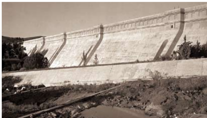
The 41 m high and 389 m long Kammanassie Dam near Oudtshoorn, completed in 1923, was one of the first large dams to be constructed under the Department of Irrigation.
