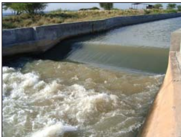
A measuring flume in the Orange-Vaal Canal.
