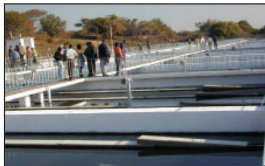
Site visit to the lolanda waterworks, Kafue river, Zambia.
