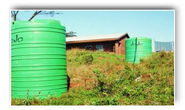
Signs of success: Two additional tanks have been erected further down the slope, to collect overflow water from the main storage tank at Tshanowa Primary School, where a fog har vesting system has been installed.
