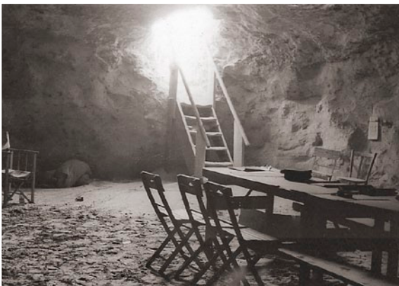
In Roman times farming was practised along the North African coastal areas. Water was stored in underground cisterns carved out of the soft limestone rock. During the war these cisterns were used by both sides as shelters from enemy bombs and shells as the battles raged backwards and forwards across Libya. The only access to the cisterns was through a wide hole in the solid roof of the cistern. This Roman cistern was converted into brigade headquarters. The large entrance was constructed by wartime engineers.
