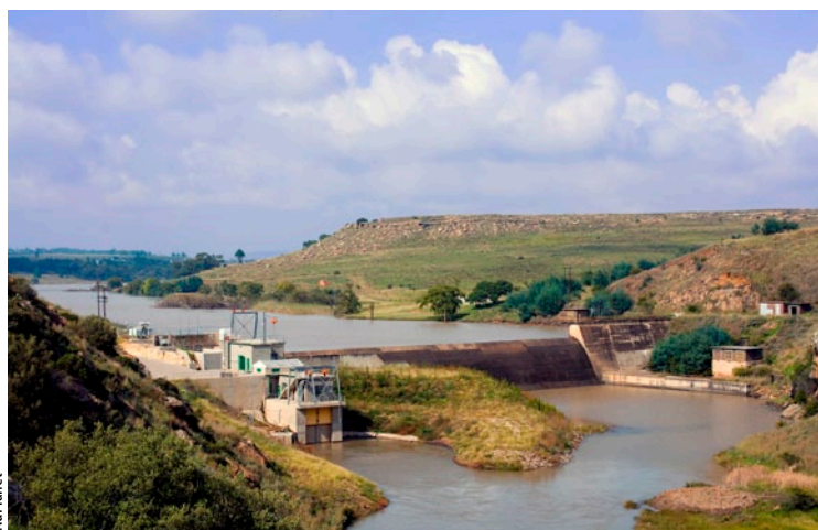
Bethlehem Hydro's 3 MW operation on the wall of the Sol Plaatje Dam.
