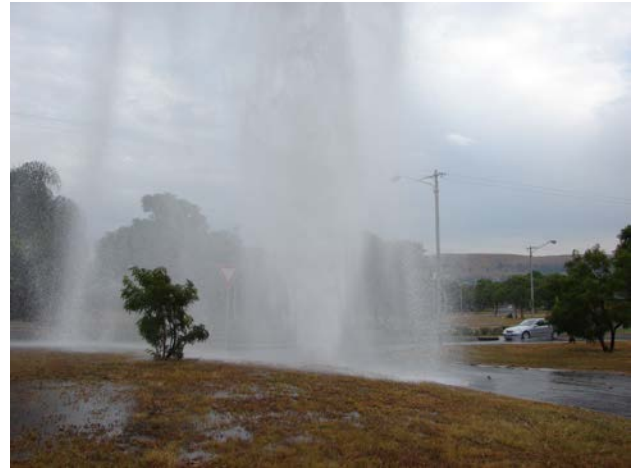
Water leaks are not always as spectacular as this burst water main, however, they present a real problem for South Africa's water service providers.
