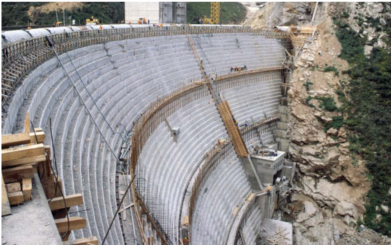
Wolwedans Dam during construction
